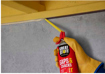
Rim Joist/Sill Plate
